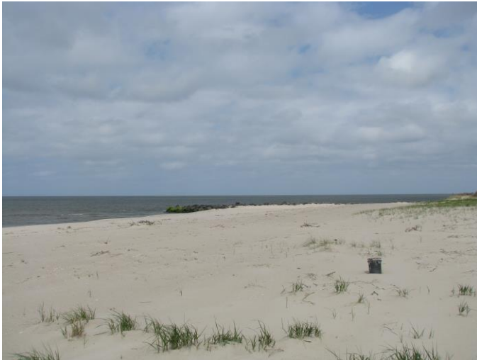
In spite of being two cells removed from direct sand placement in 2011, this cell has gained sand on the dune and beach with little change offshore as longshore drift moved sand west filling behind the terminal groin.
