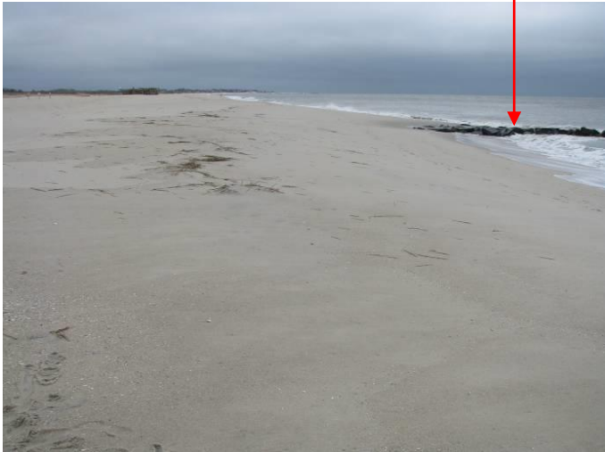
The photo taken on April 2013 the cell is completely filled with sand added to the berm elevation burying most of the exposed groin rock at the beachface.
