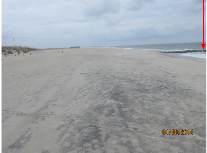
Taken on April 8, 2014 this photo shows beachface erosion has exposed more of the rocks along the shoreline. Note the positions of the red arrows in each photo.
