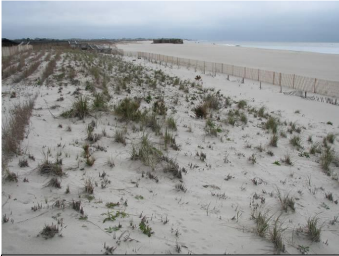
By April 2013 a new row of fencing was added seaward of the partially buried row present earlier. The berm elevation was higher and further seaward than a year earlier.
